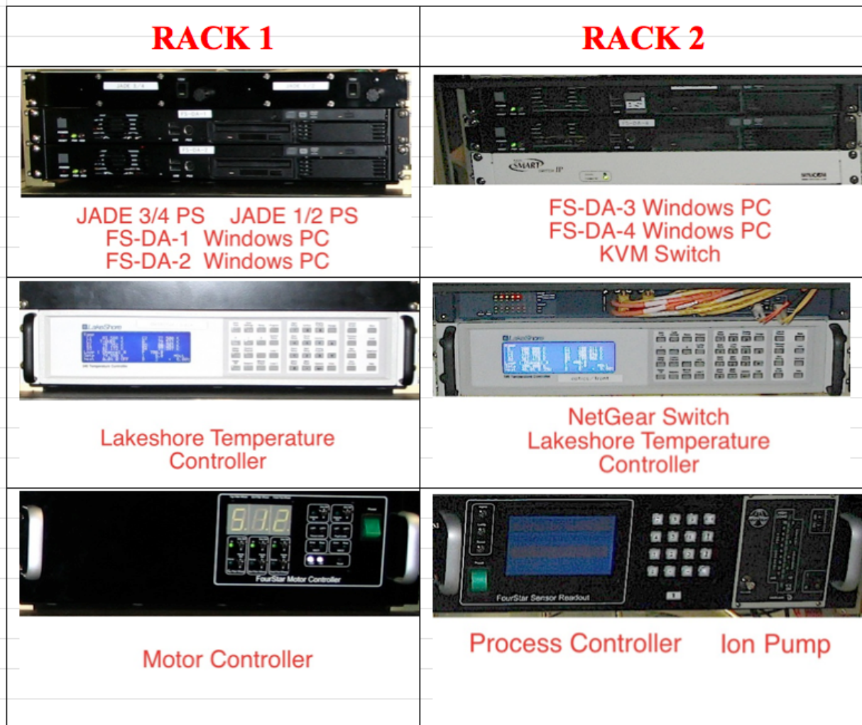
Figure 2. Electronics chassis in the 2 racks.
