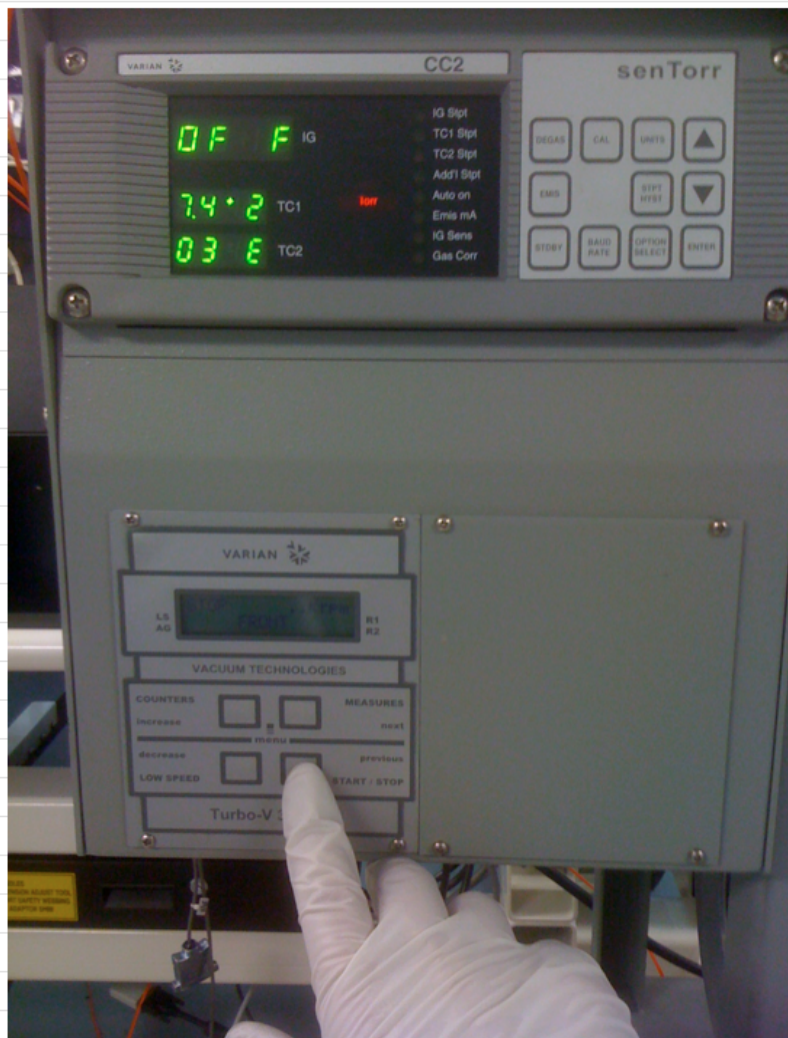
Figure 5. Turbo-pump control panel.
